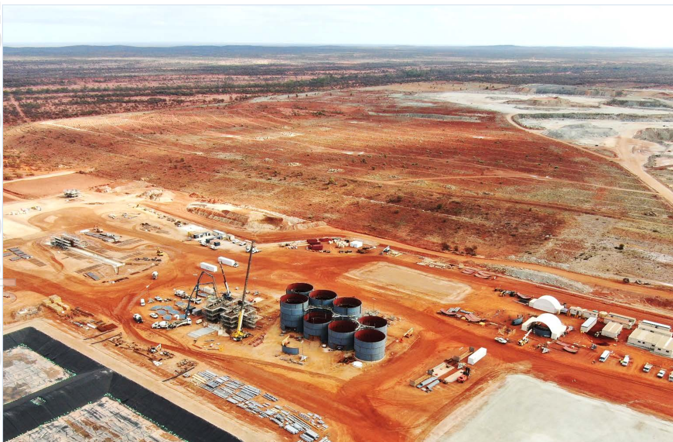
Figure 1: A two-day concrete pour of the mill plinths is being completed on 1 July 2021 and four of the eight CIL tanks are now at full height. Substantial steel deliveries are now on site, along with all major long-lead items in anticipation of the next key phase of steel-erection.
